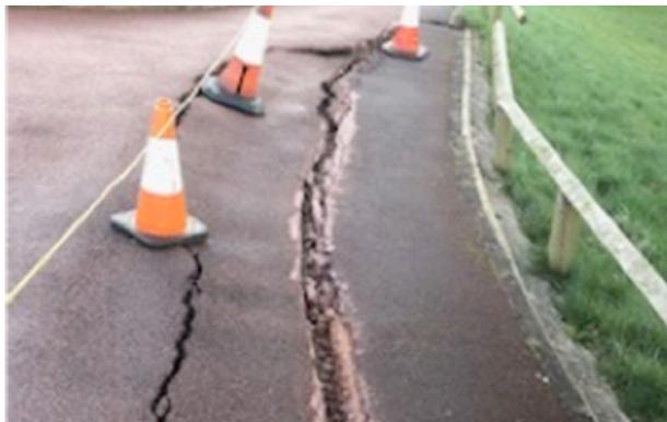
Earth Environmental were requested to assess the stability of a slope by the 18th green. For a number of years there was slippage of the footpath at the top of the slope.
